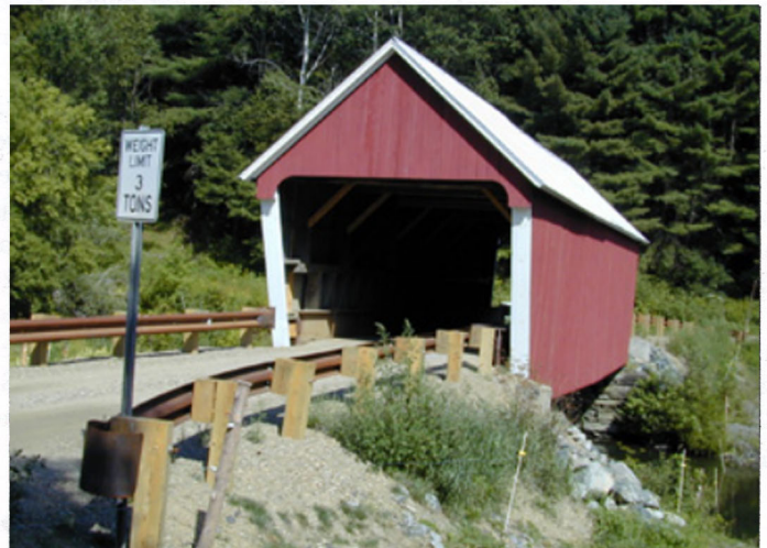
Gifford Bridge in Town of Randolph. Photo by Joe Nelson, August 15, 2001
