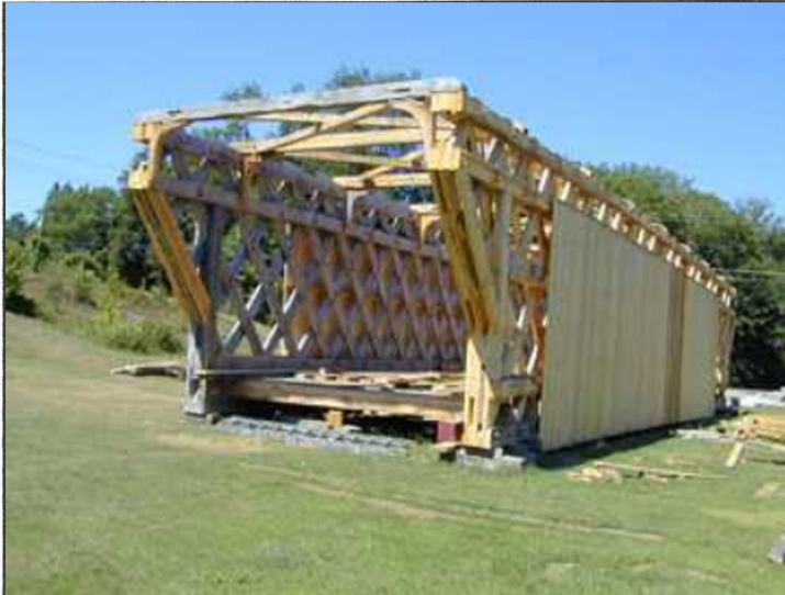
North Hartland Bridge under construction by Jan Lewandoski. Photo by Joe Nelson, August 15, 2001
