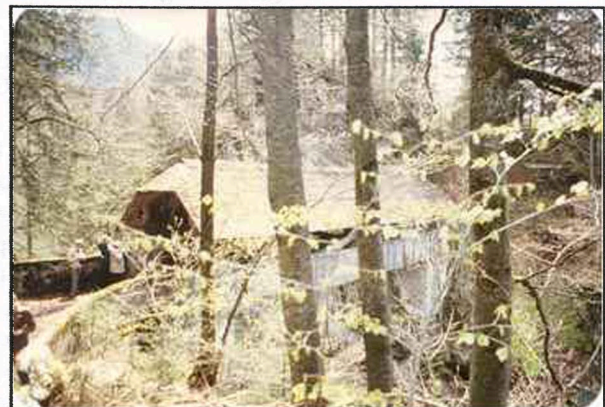
Montbouvon Bridge- 1667 WGN S-07-03
