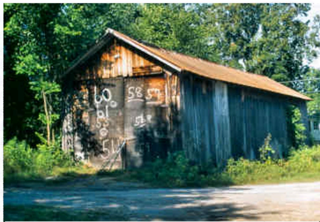
Twin Bridge, Rutland, VT 45-11-10 Photo by Joe Nelson 1997
