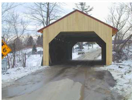
Maple Street Bridge, Fairfax, VT
