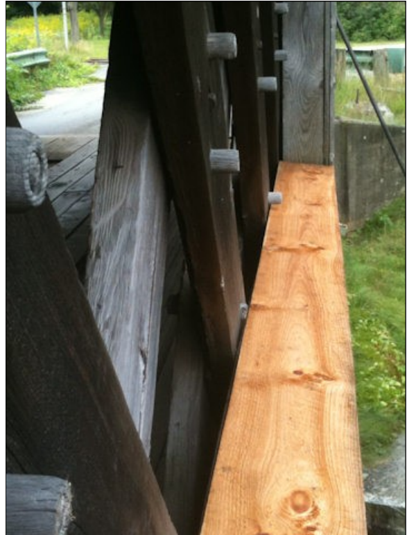
Bartonsville window sill repairs—August 2011
