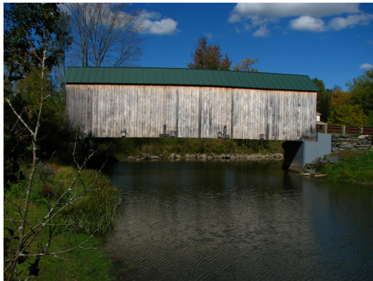
East Fairfield Bridge
