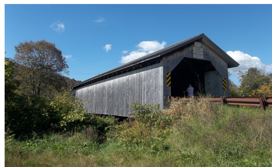
Hopkins Bridge, Enosburg
