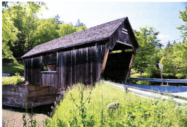
Warren Covered Bridge - Photo by DuBois & King, Inc.
