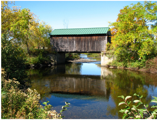
Scribner Bridge, Johnson
