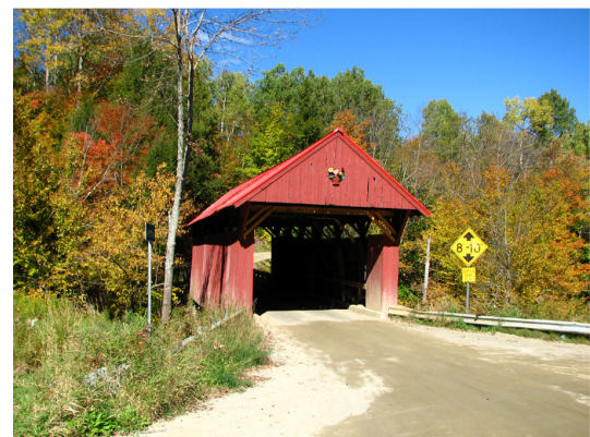
Red Bridge, Morristown
