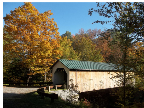
Hutchins Bridge, Montgomery
