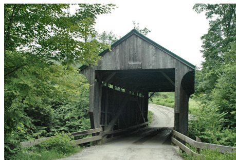
Coddington Hollow Bridge, Waterville
