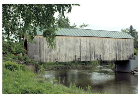
East Fairfield Bridge
