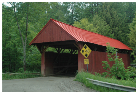
Red Bridge, Morristown
