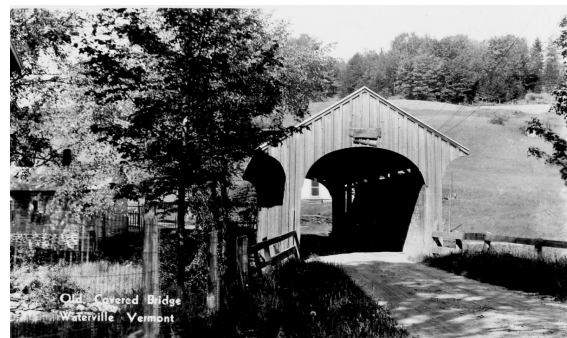
Church Street Bridge, Richard E. Roy Collection
