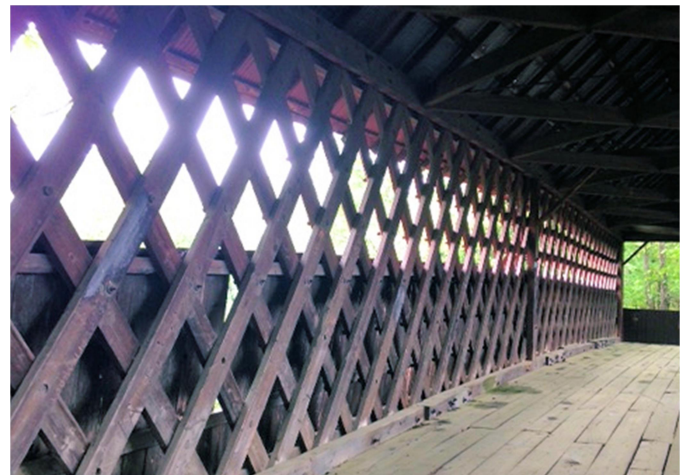
Pont de la Frontiere, near Mansonville, Quebec, 1896
