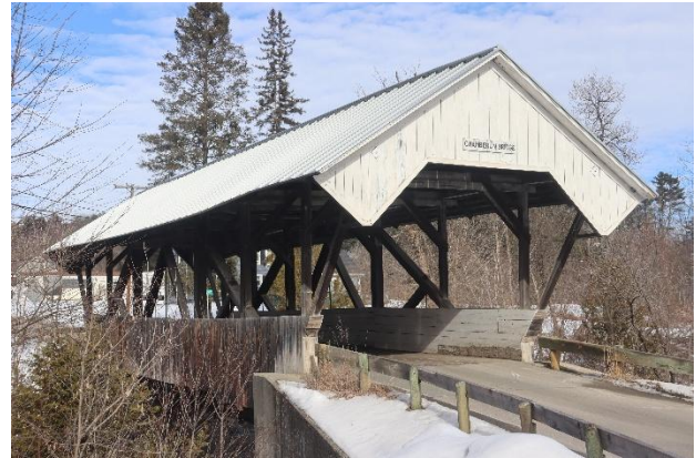
Chamberlin Covered Bridge - Photo by Mark Maddox
