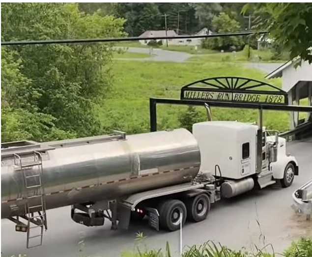
A tractor trailer being stopped by new crash barriers at the Miller's Run Covered Bridge.
