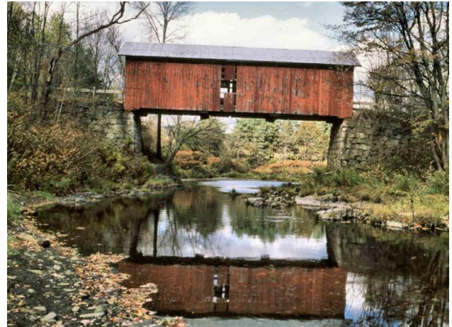
Slaughterhouse Covered Bridge - photo by Joe Nelson
